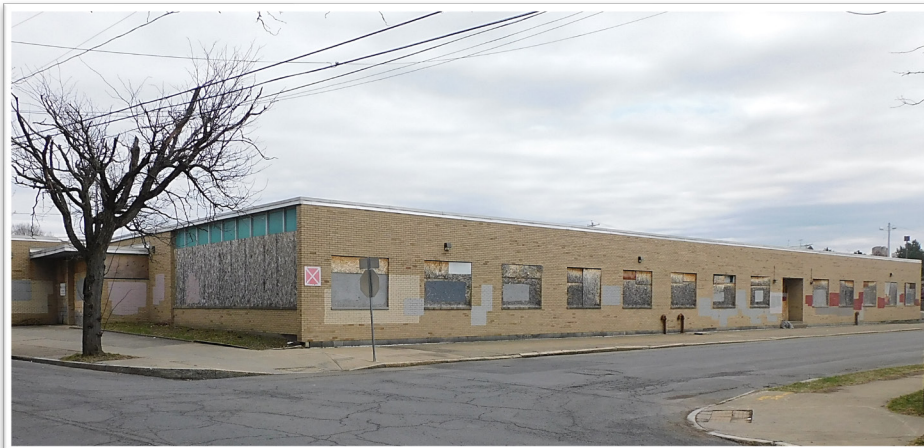
Top: The project site was assembled by the Land Bank and comprises approximately 1.86 acres in the heart of Albany, New York.
